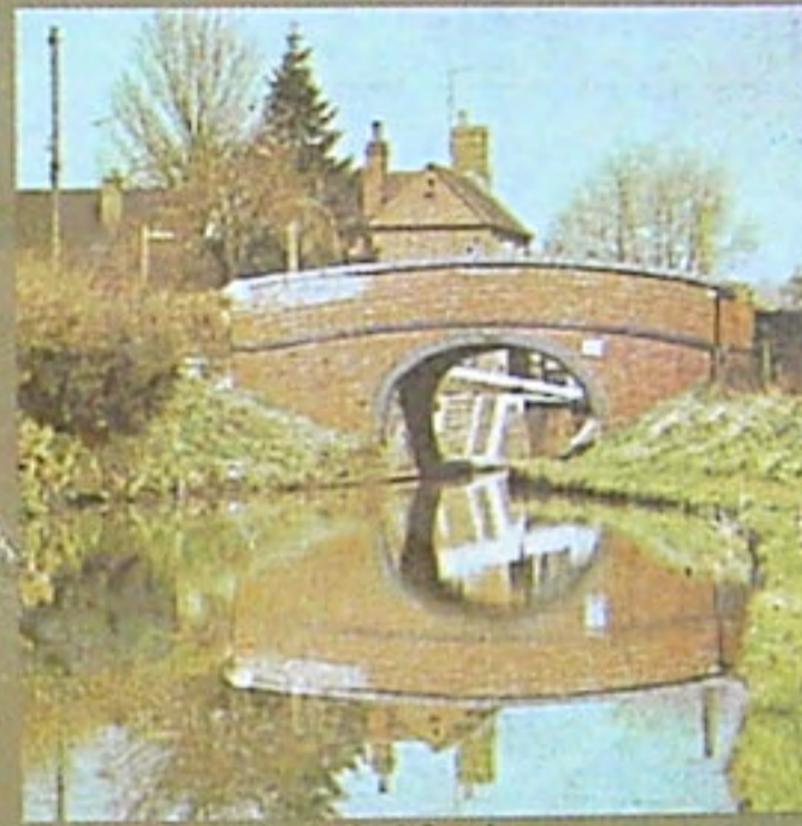
Bridge at Cropredy, Oxford Canal
