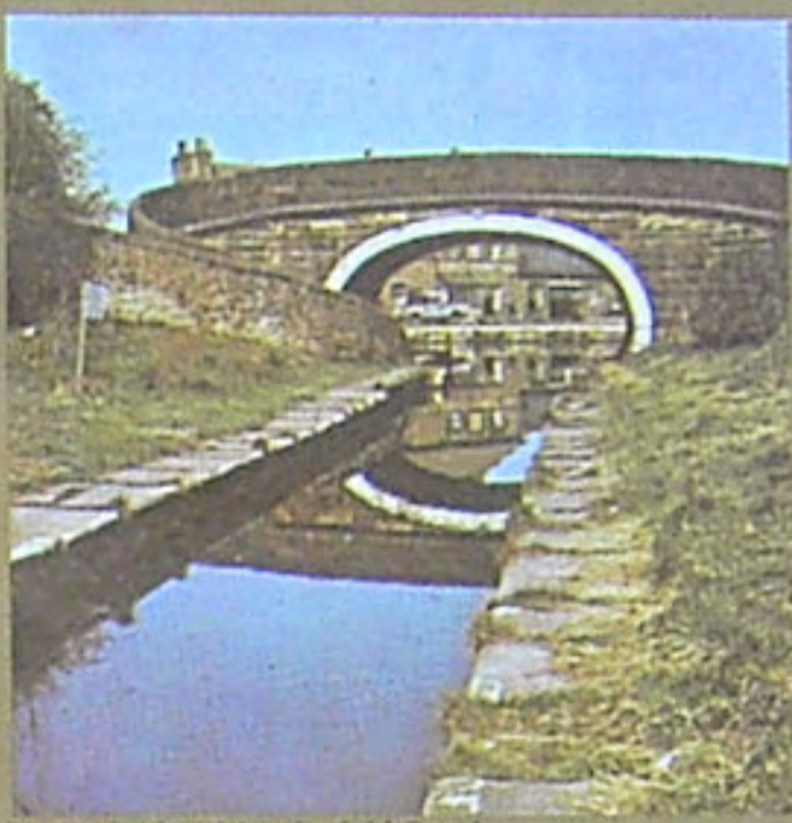
Roving bridge, Macclesfield Canal
