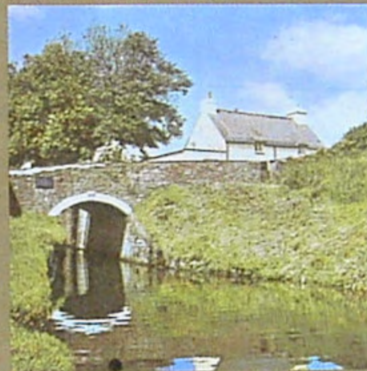
Cefn Brynich Bridge, Monmouthshire & Brecon Canal
