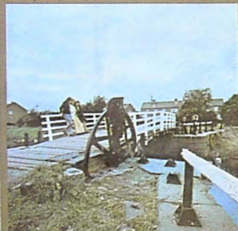
Bascule bridge, Forth & Clyde Canal
